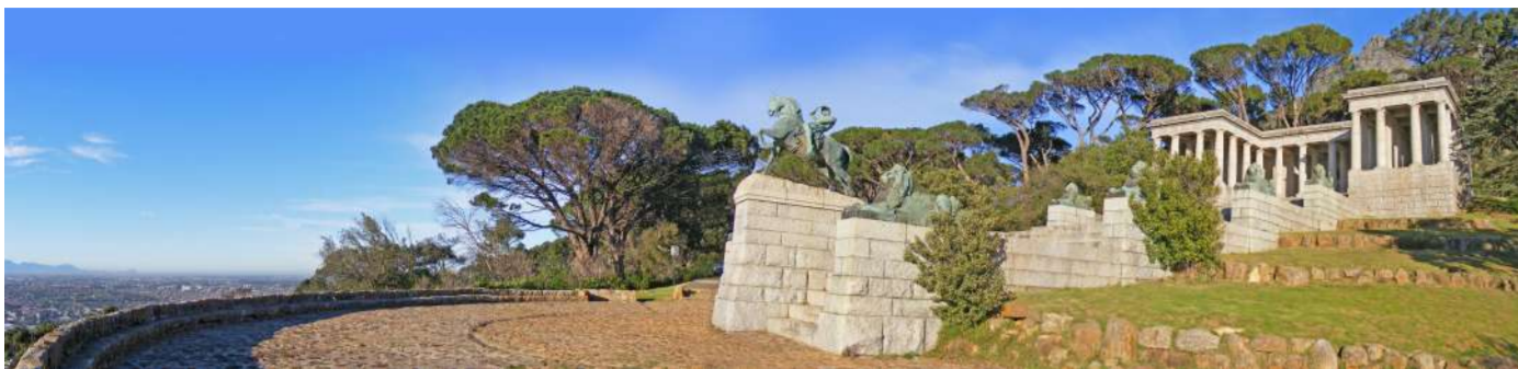
Rhodes Memorial is made up of three sections. The first is a semi-circular terrace of embedded sandstone cobbles. From here, one ascends the 49-step terraced steps which flank the statue of Physical Energy and the avenue of eight bronze lions. The last section is a U-shaped modernised Doric temple. This section contains 38 columns. The pedestal with Rhodes' bust is situated in the centre in a shallow recess.
