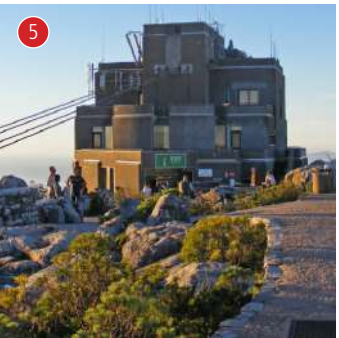
Upper Cableway Station
