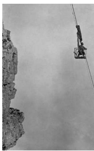
An early cableway used in the construction of the reservoirs in the late 1800s
