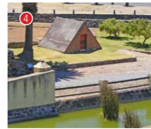
4 The Ravelin was added in 1697 just after the new entrance and Bell Tower were moved to this position. The idea behind the Ravelin was the concept of 'defence in depth'. The entrance road angles right which does not allow an enemy a direct shot at the entrance gate.
