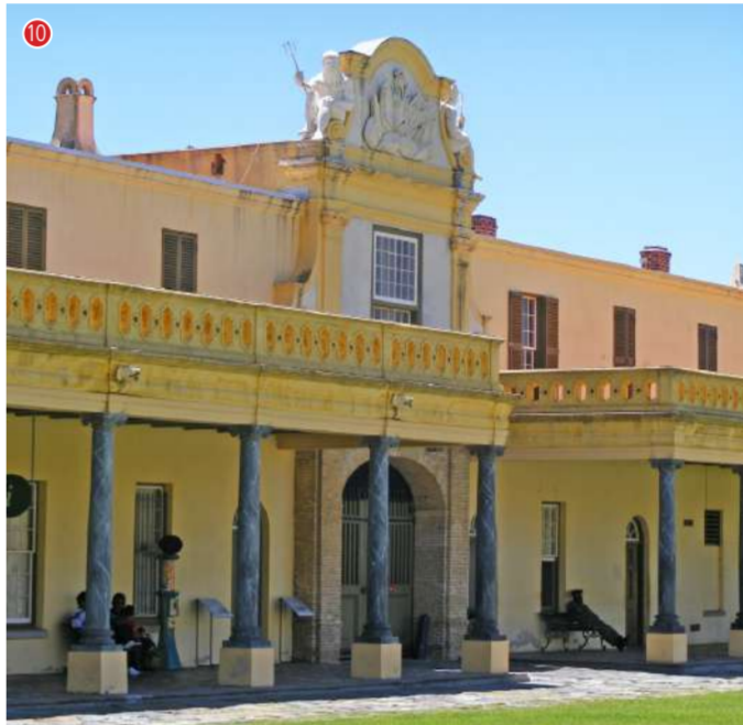
View of the Inner Gable, showing the iron pillars (painted to look like marble) which replaced the original wooden pillars. The remodelled sculpted figures can be seen on either side of the gable.
