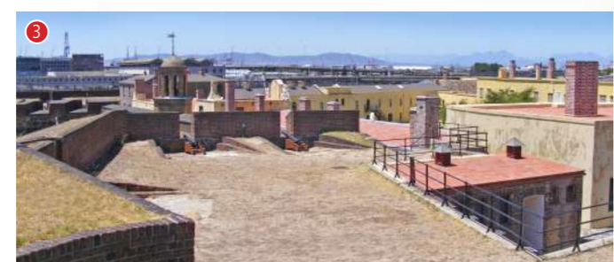
3 A view from Leerdam Bastion. This bastion and Oranje are higher than the bastions on the seaward side, allowing gunners from these positions to shoot over the seaward bastions.
