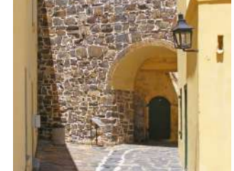
2 A visible section of Van Rhee's cross-wall which runs from Catzenellenbogen Bastion to mid-point of the curtain wall between Leerdam and Oranje. This wall was built to make an inner and outer court for a better defensive solution.
